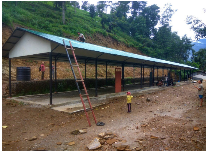
The school building under construction. The roof has skylights for each of the classrooms. The walls, windows and doors are currently being installed.
